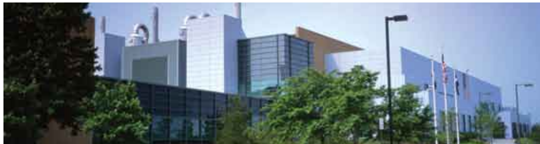
Micron Technology, Inc.'s Manassas, Virginia facility
